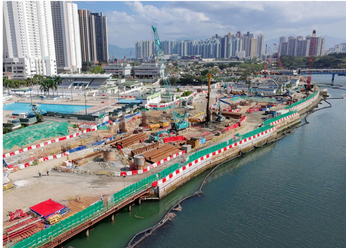
Existing Site Condition of MTRCL Site
